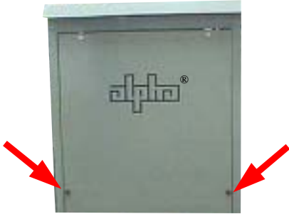
Figure 4-1; Security Bolt Location
