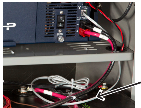
Fig. 3-17, XM3 Series Precision Temperature Sensor (PTS) Placement
