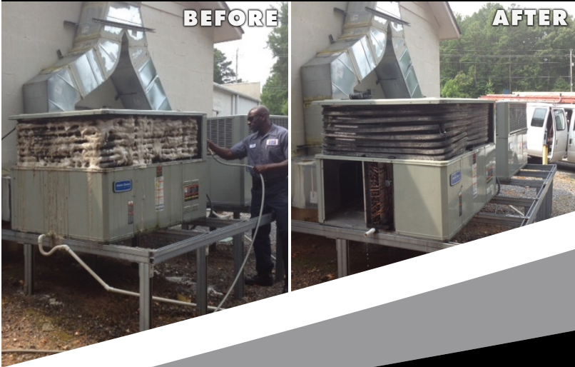
Routine HVAC maintenance prevents costly repairs and helps maintain an ideal operating environment for critical facility equipment.
